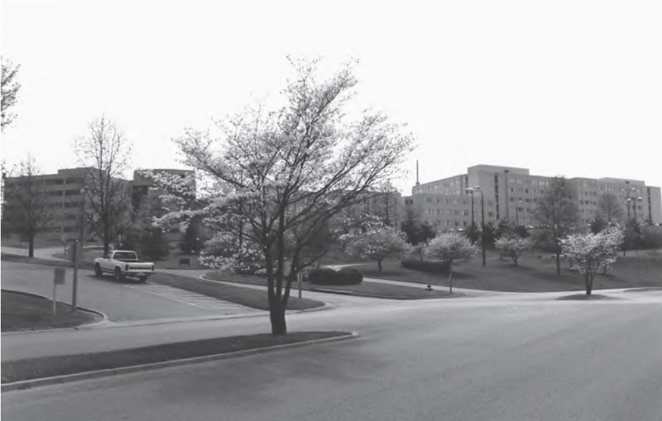
The United States has approximately 5,700 hospitals employing more than 6 million workers. Physician-owned clinics (like the one pictured to the left in the photo) often locate adjacent to hospitals (pictured on the right).
